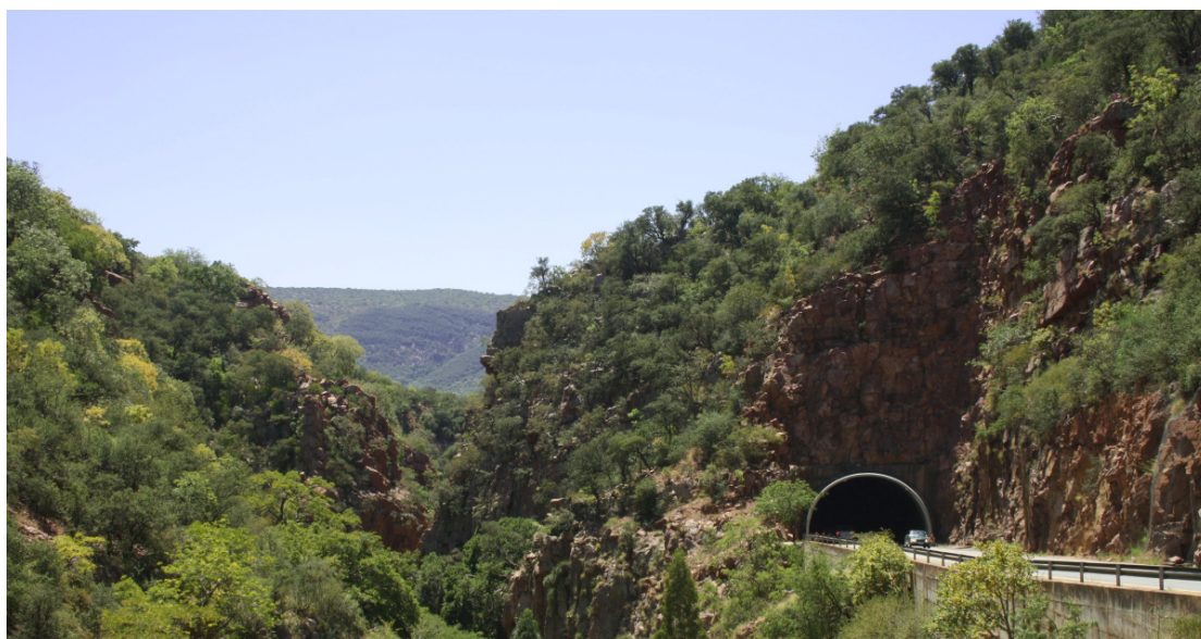
Figure 7.4: Cliffs and valleys of the Soutpansberg, with the Hendrik Verwoerd tunnel.
