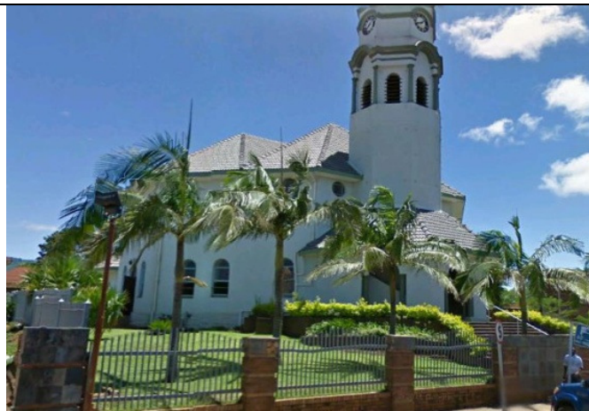
Figure 7.36: Buildings found in the urban environment.
